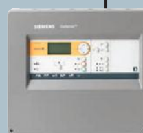
Fire control panel conventional FC120
